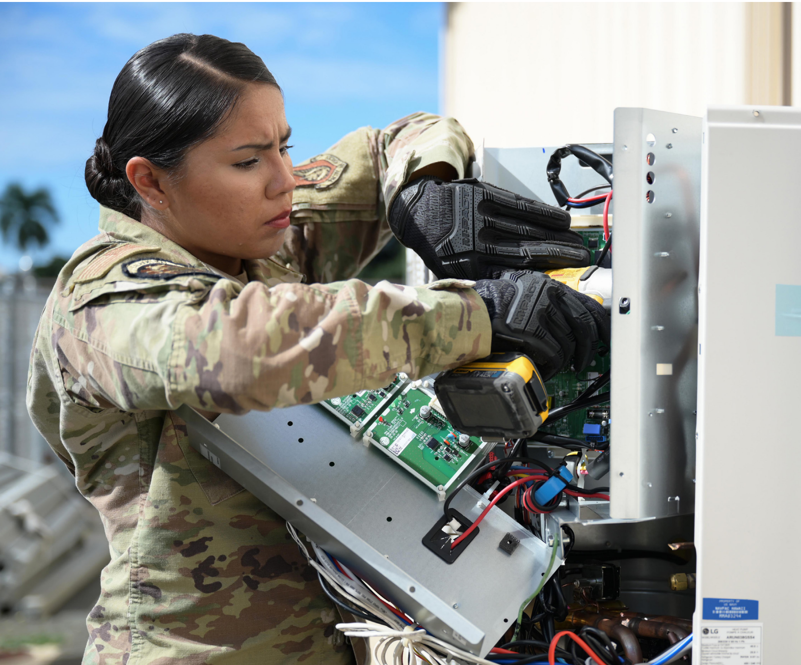
Air Force Airman 1st Class Lorraine Tulee prepares an HVAC unit for a circuit board replacement at Joint Base Pearl Harbor-Hickam, Hawaii, Feb. 25, 2025. (Air Force Staff Sgt. Alan Ricker)
